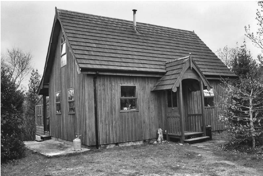
Figure 1.2 Locals thought this blow-in carpenter ‘mad’ to construct a wooden house in such a gale-swept area as County Clare, west Ireland. More than a decade later, the house still stood, in good shape.
